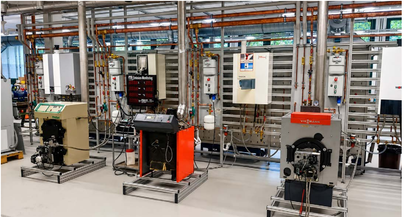
Combined workstation with energy supply and drainage column for wall- and floor-standing heat generators
