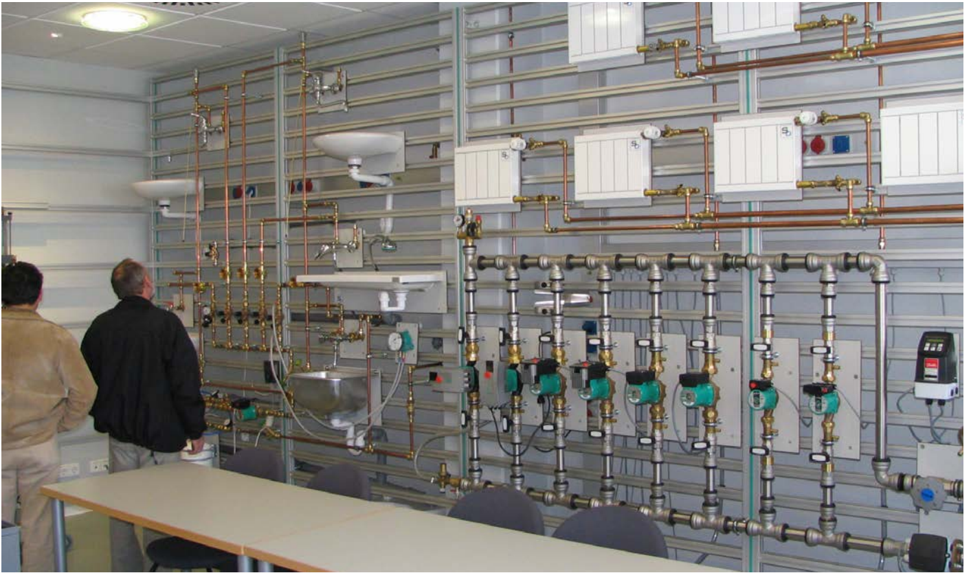
Technical training room
